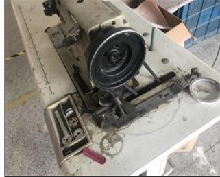
Photo of non-conformity NC-The sewing machine was not equipped with belt guard.JPG
