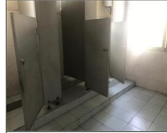
Photo of the sanitary facilities Toilets.JPG
